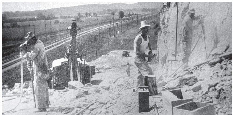
► Workers construct Route 66 near Allenton in the 1930s. // Courtesy of the Eureka Historical Society
